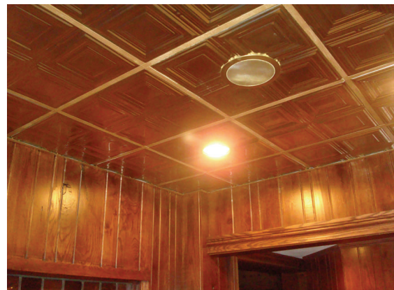
Tin ceiling in the main lobby
