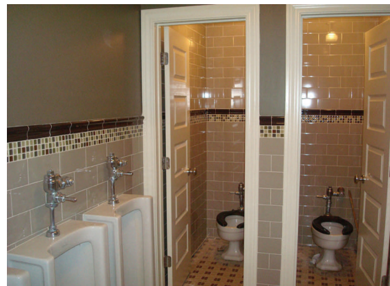
Completely remodeled bathrooms
